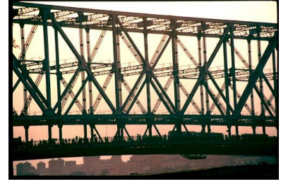
Figure 6.6: The Howrah bridge. Trusses are such a good idea that they are used recursively. The bars in some large trusses, like this one or the Eiffel Tower, are themselves made of trusses (courtesy Bipin Chandra, www.bipinchandra.co.uk ).
