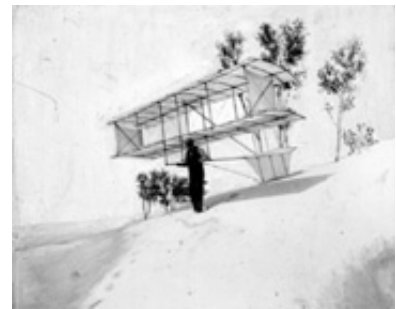
Figure 5.3: Chanute Glider, 1897. The Wright brothers' first planes were near copies of the 4-wing gliders built a few years earlier by Octave Chanute. Chanute was a retired bridge designer. Structurally these early biplanes were essentially flying bridges. The Wright brothers were preoccupied with trusses. Their first inspiration and main airplane patent was about how to control the distortion of a truss ('wing warping'). The Wrights even thought of the threads in their wing fabric as bars in a truss. Take away the outer skin from many small modern planes and you will also find trusses. (National Air and Space Museum Negative 1A-2036084-10697)
