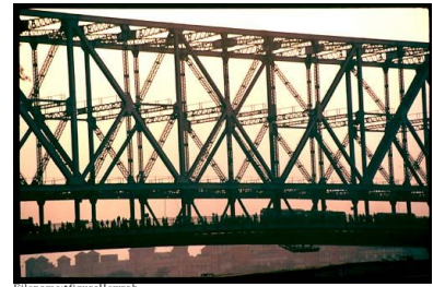
Figure 5.6: The Howrah bridge. Trusses are such a good idea that they are used recursively. The bars in some large trusses, like this one or the Eiffel Tower, are themselves made of trusses (courtesy Bipin Chandra, www.bipinchandra.co.uk ).
