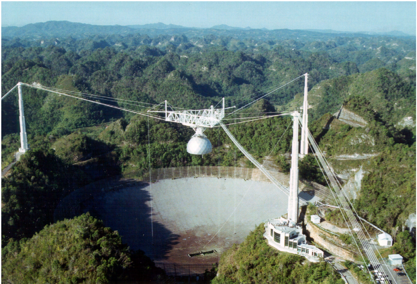
Figure 4.7: “Suspended 450 feet above the reflector is the 900 ton platform. Similar in design to a bridge, it hangs in midair on eighteen cables, which are strung from three reinforced concrete towers. One is 365 feet high, and the other two are 265 feet high.” Courtesy of the NAIC-Arecibo Observatory, a facility of the NSF.
