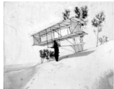
Figure 5.3: Chanute Glider, 1897. The Wright brothers first planes were near copies of the planes built a few years earlier by Octave Chanute, a retired bridge designer. Structurally these early biplanes were essentially flying bridges. The Wright brothers were pre-occupied with trusses. Their first inspiration and main airplane patent was about how to control the distortion of a truss ('wing warping'). The Wrights even thought of the threads in their wing fabric as bars in a truss. Take away the outer skin from many small modern planes and you will also find trusses. (National Air and Space Museum Negative 1A-2036084-10697)
